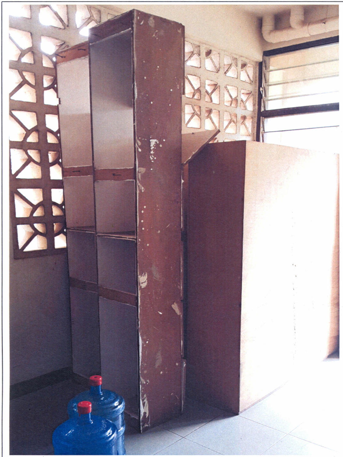
Fig. 1. A Picture Showing Cupboards Left Near Back Entrance Door To The Main Building
