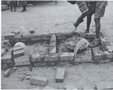
Fig. 10a Adding bricks to raise the foundation
