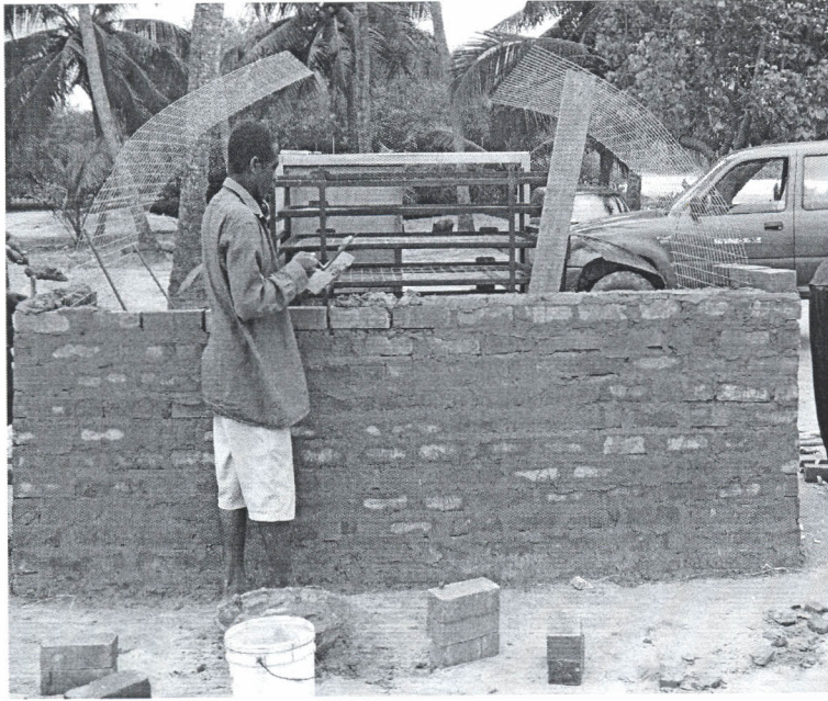
Fig. 27 Laying of bricks (back of oven)
