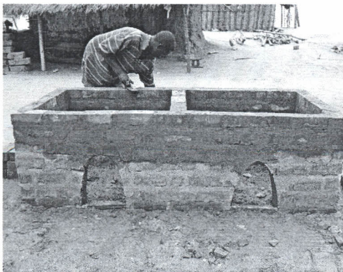
Fig. 11a The completed brick work of the chorkor oven
