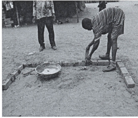
Fig. 9b Laying of the foundation
