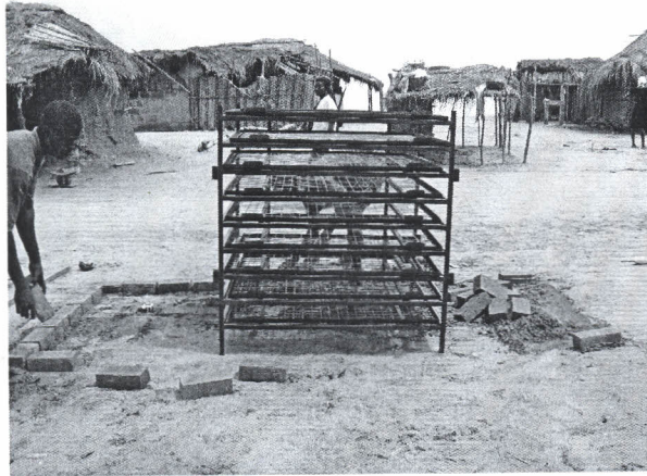
Fig. 22 Laying of foundation and positioning of metal frame
