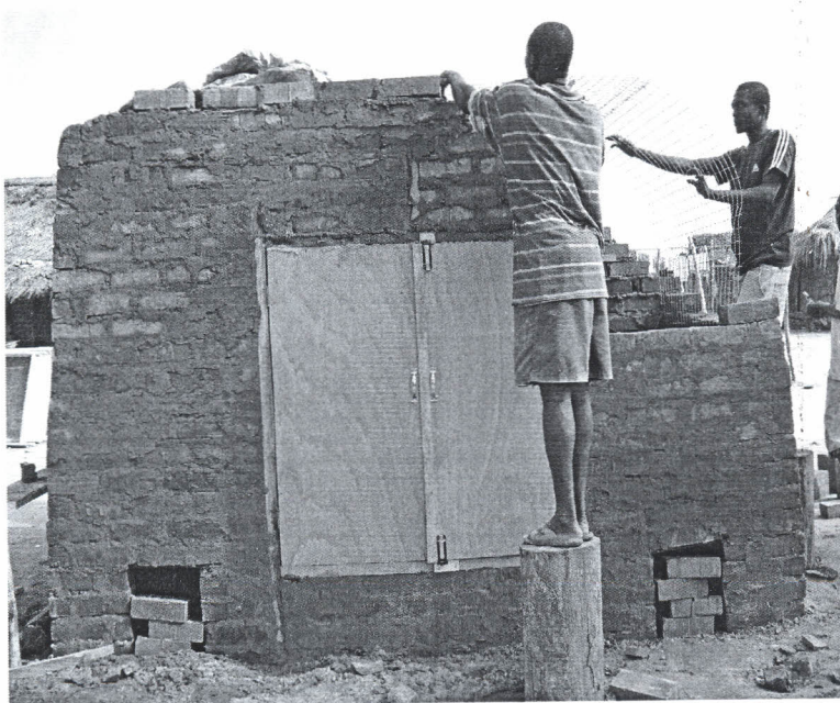
Fig. 28 Laying bricks on top of door frame
