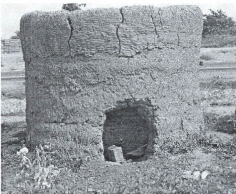
a. Round oven with single round stokehole
