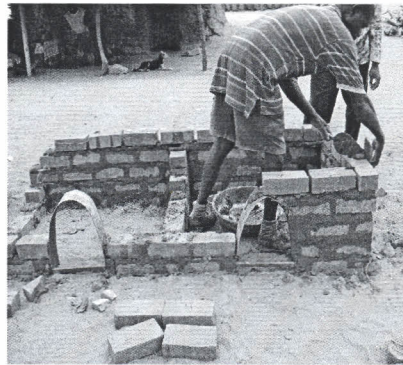
Fig. 10b Leveling of layers of bricks
