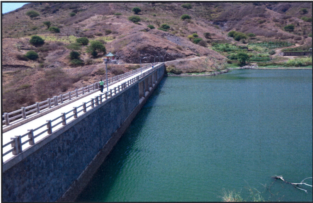
Figure 25. Newly constructed dam for irrigated farm fields
