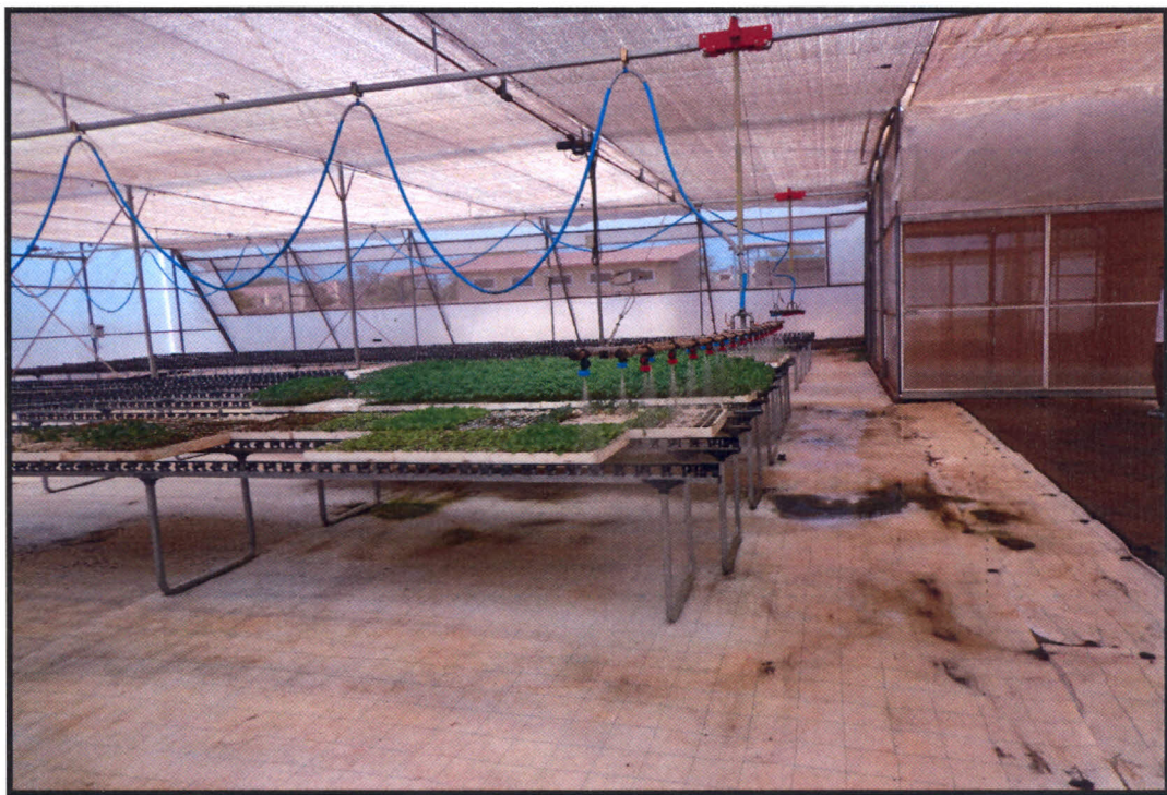
Figure 19. Automated watering of hydroponics nursery
