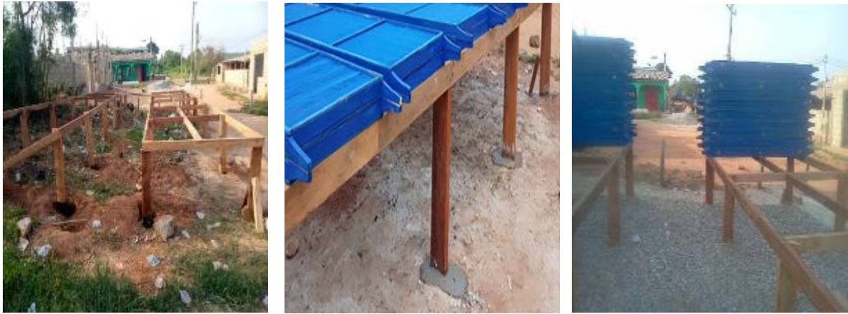
Fig 7. Construction of platform and drying racks at Moree
