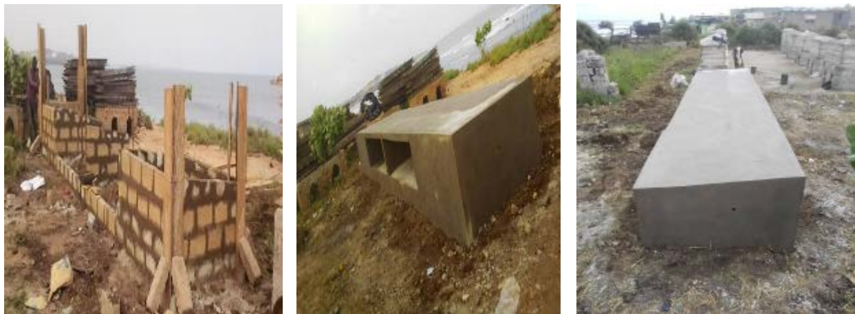
Fig 6. Construction of concrete drying platform at Tema New Town
