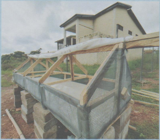
A solar tent for drying was introduced and constructed for the group
