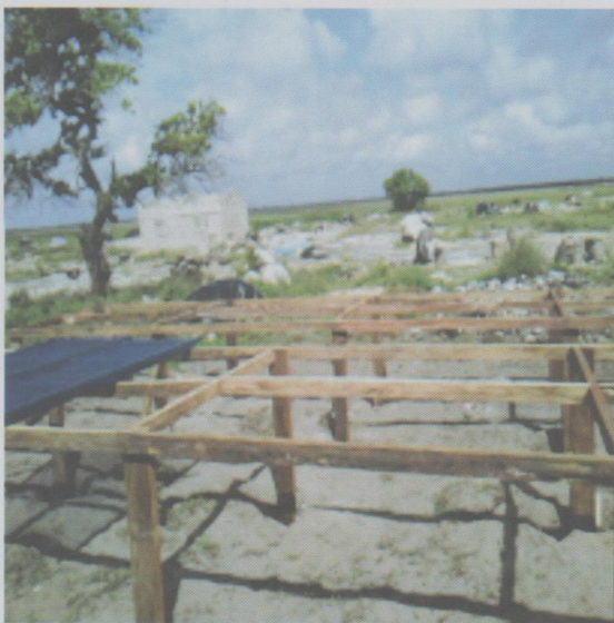
Construction of drying platforms
